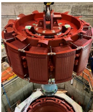
Ogamigo Hydroelectric Power Station (installing the new generator rotor)
